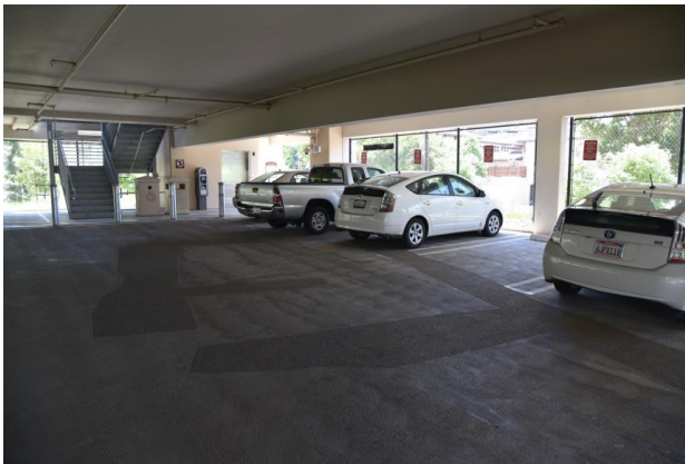
Figure 16 Native Dormitory Outline in Concrete
